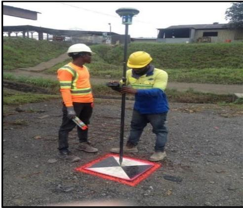
**Fig. 6 Survey of Ground Control Point**
