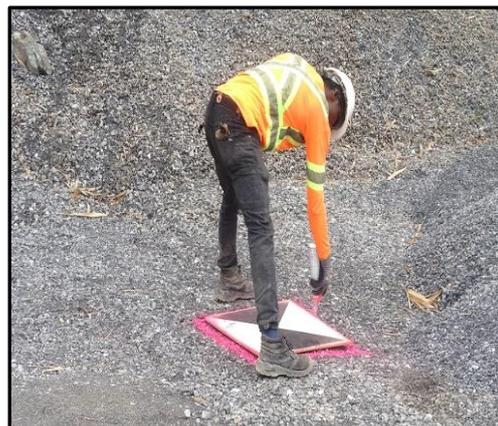
**Fig. 5 Establishment of Ground Control Point**
